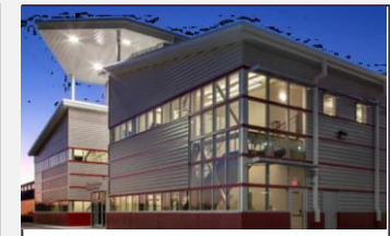
Corrosion testing at pressures and fluid chemistry of disposal depths, at Halliburton facility in Carrollton, TX
